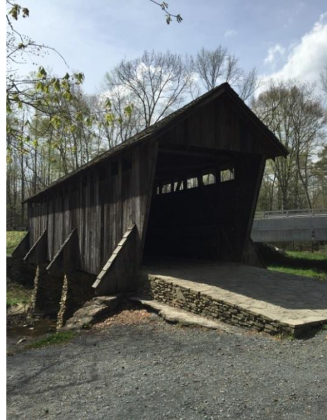
Figure 4. Pisgah Covered bridge outside Asheboro; 1 of 2 remaining covered bridges in NC
